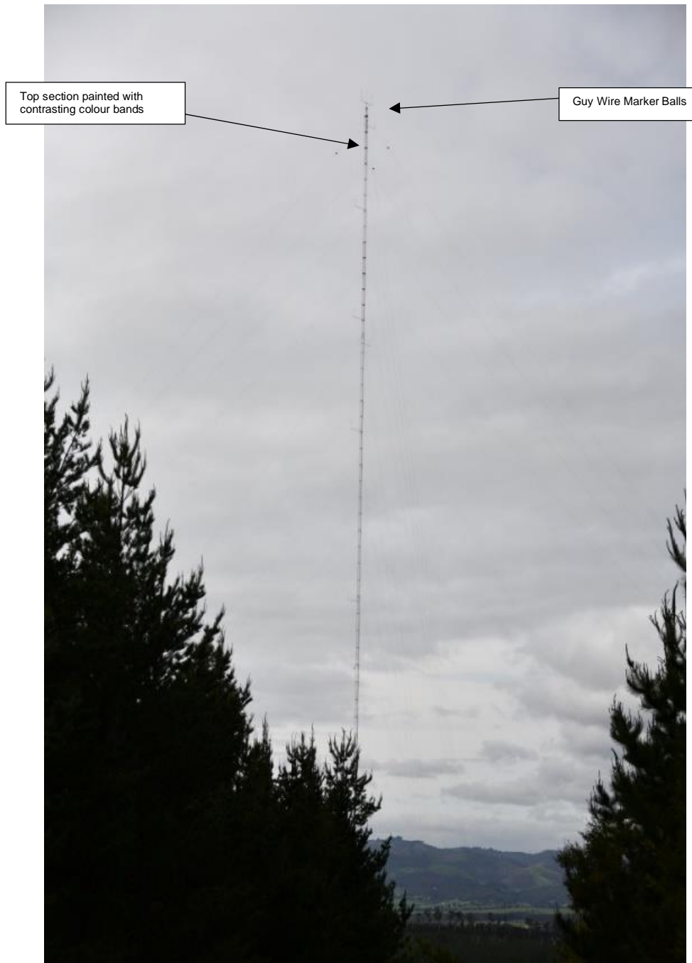
Figure 8 – A Meteorological Monitoring Mast
