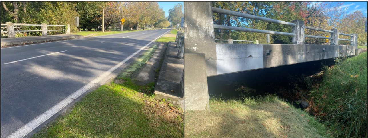
Figure 1-13 Site No. 4 – Inspection Images
