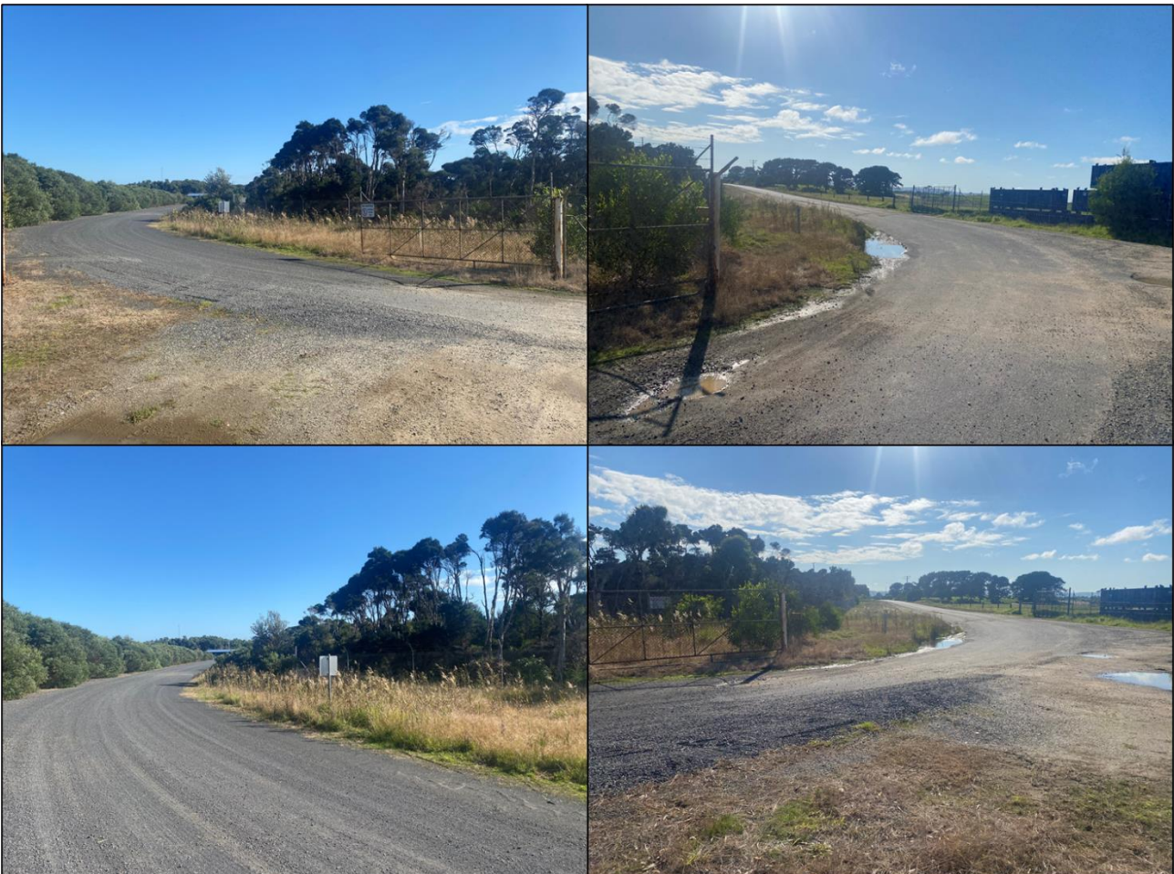
Figure 1-7 Site No. 1 – Inspection Images
