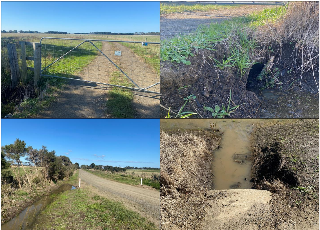
Figure 1-32 Site No. 12 – Inspection Images
