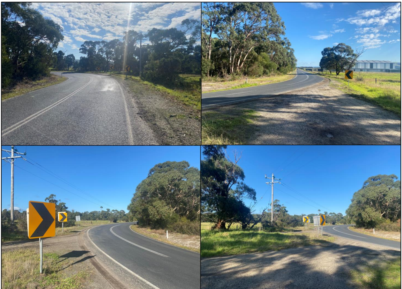
Figure 1-9 Site No. 2 – Inspection Images
