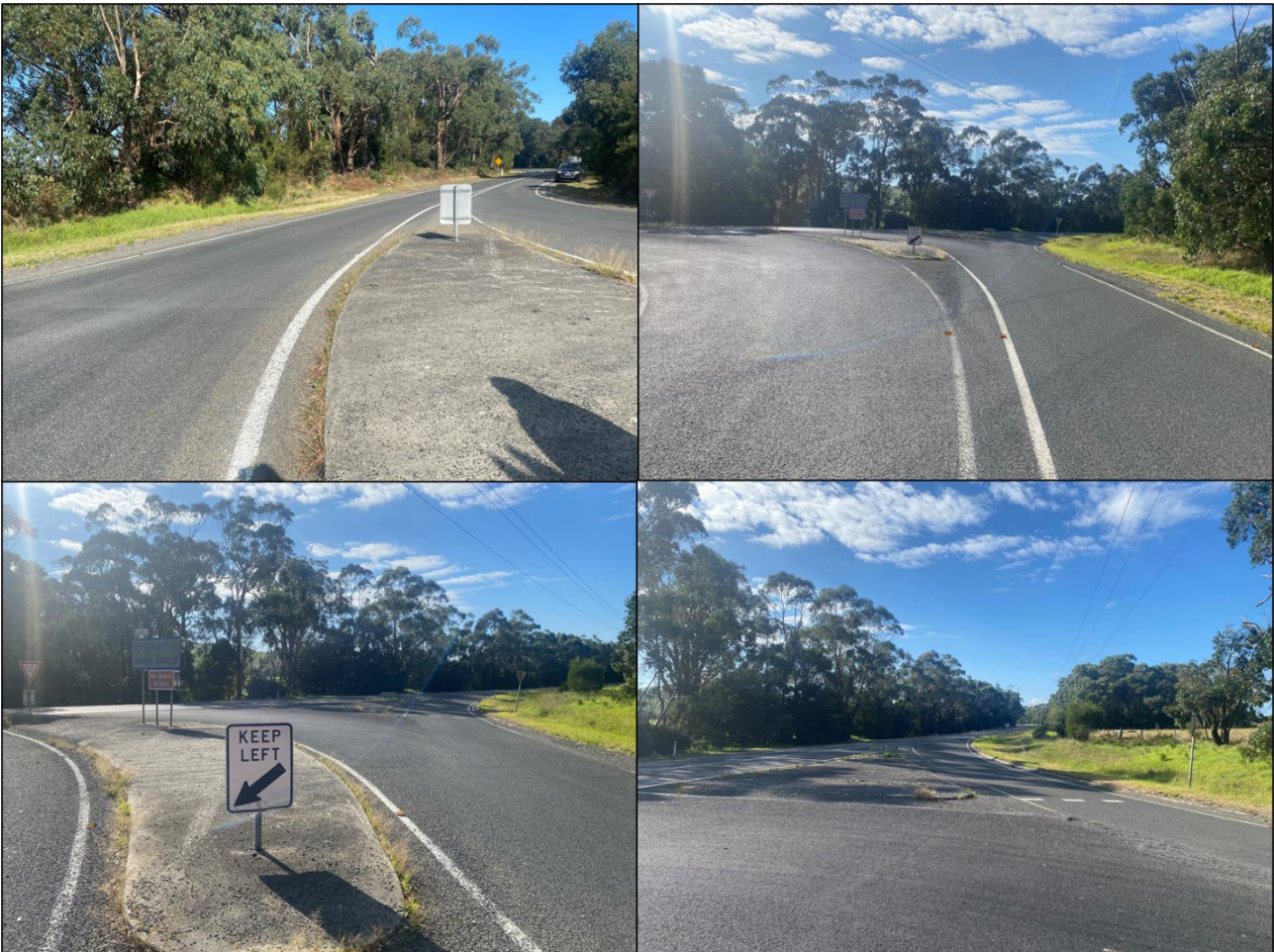
Figure 1-11 Site No. 3 – Inspection Images
