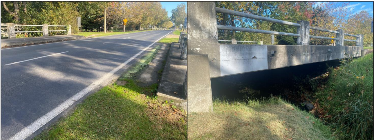
Figure 1-13 Site No. 4 – Inspection Images
