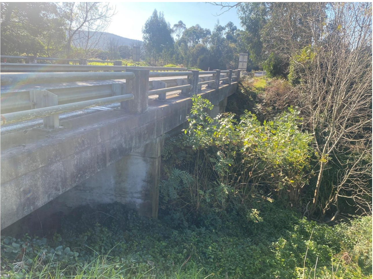
Figure 1-15 Site No. 5 – Inspection Images
