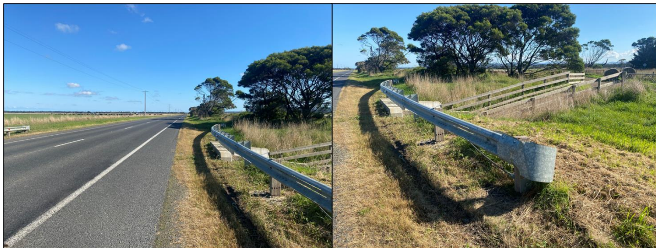
Figure 1-26 Site No. 9 – Inspection Images
