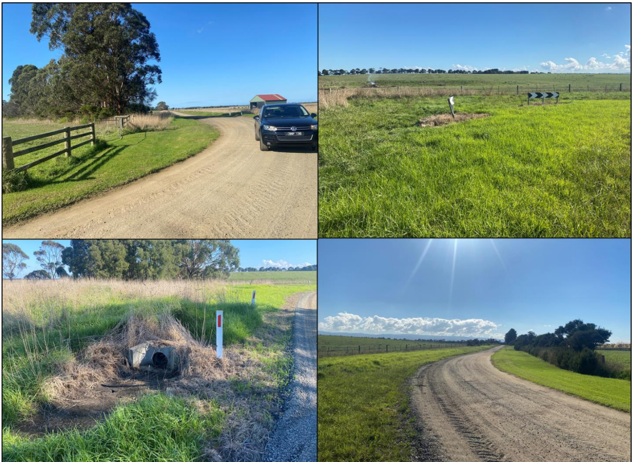
Figure 1-30 Site No. 11 – Inspection Images
