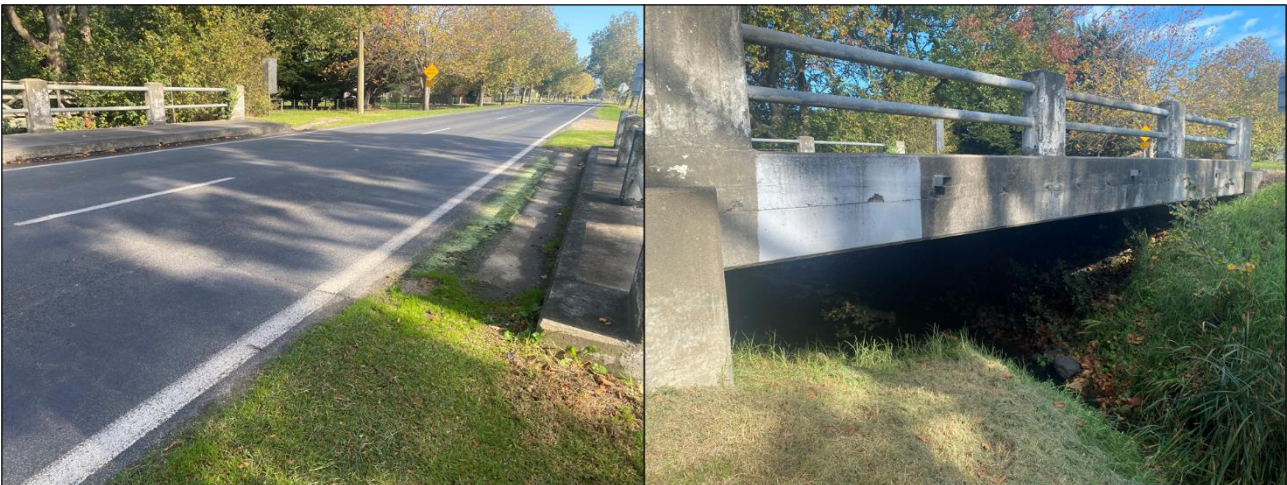
Figure 1-13 Site No. 4 – Inspection Images
