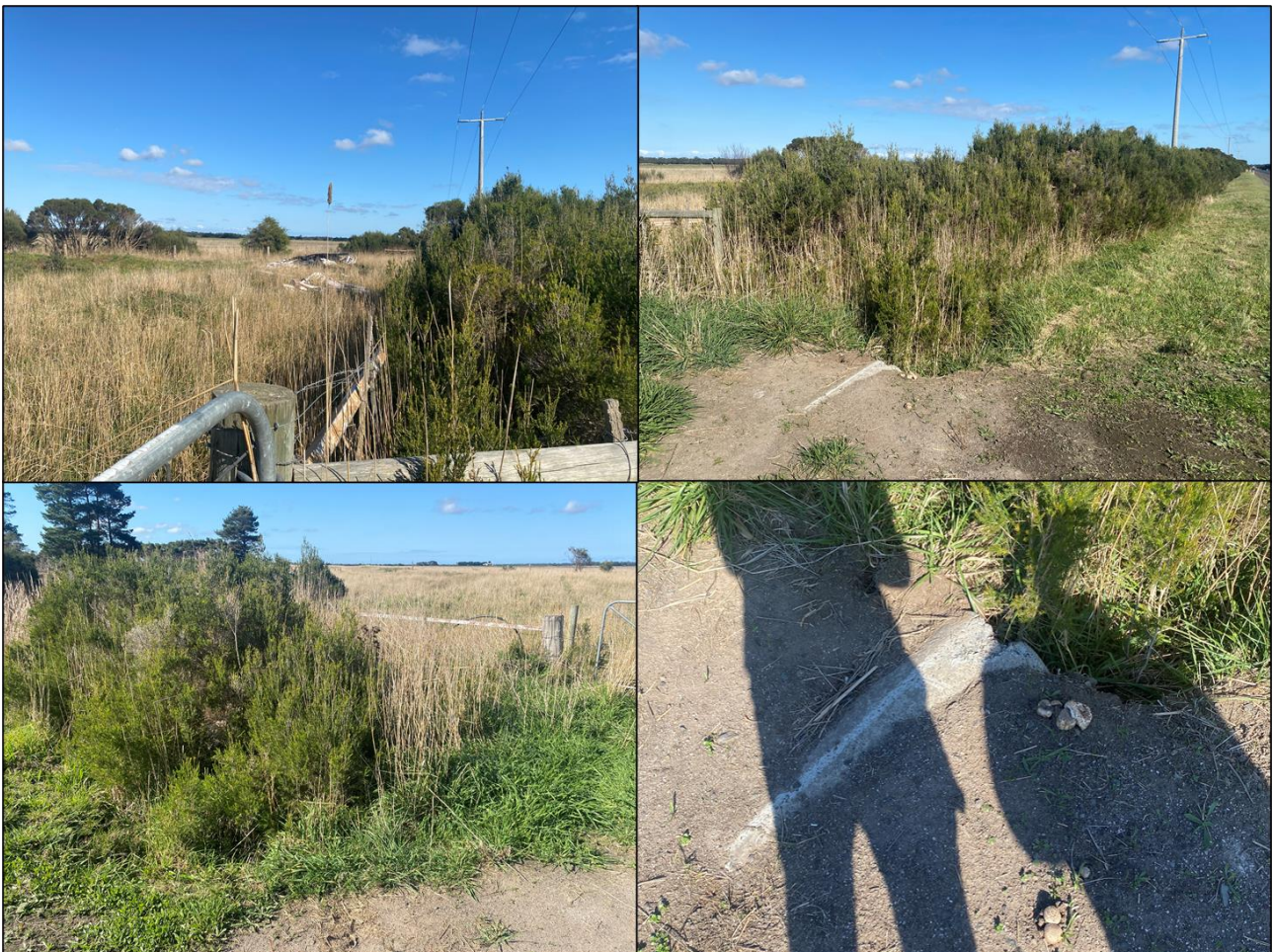
Figure 1-21 Site No. 7 – Inspection Images
